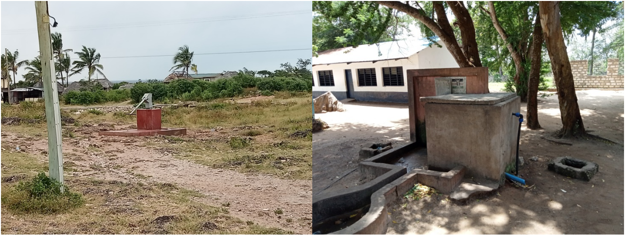
Picture vi: All schools have such boreholes that have been converted to pump water to toilets for flushing and hand washing. However, some pumps need repair or re-plumbing. Dongokundu's borehole water is too salty to use.
