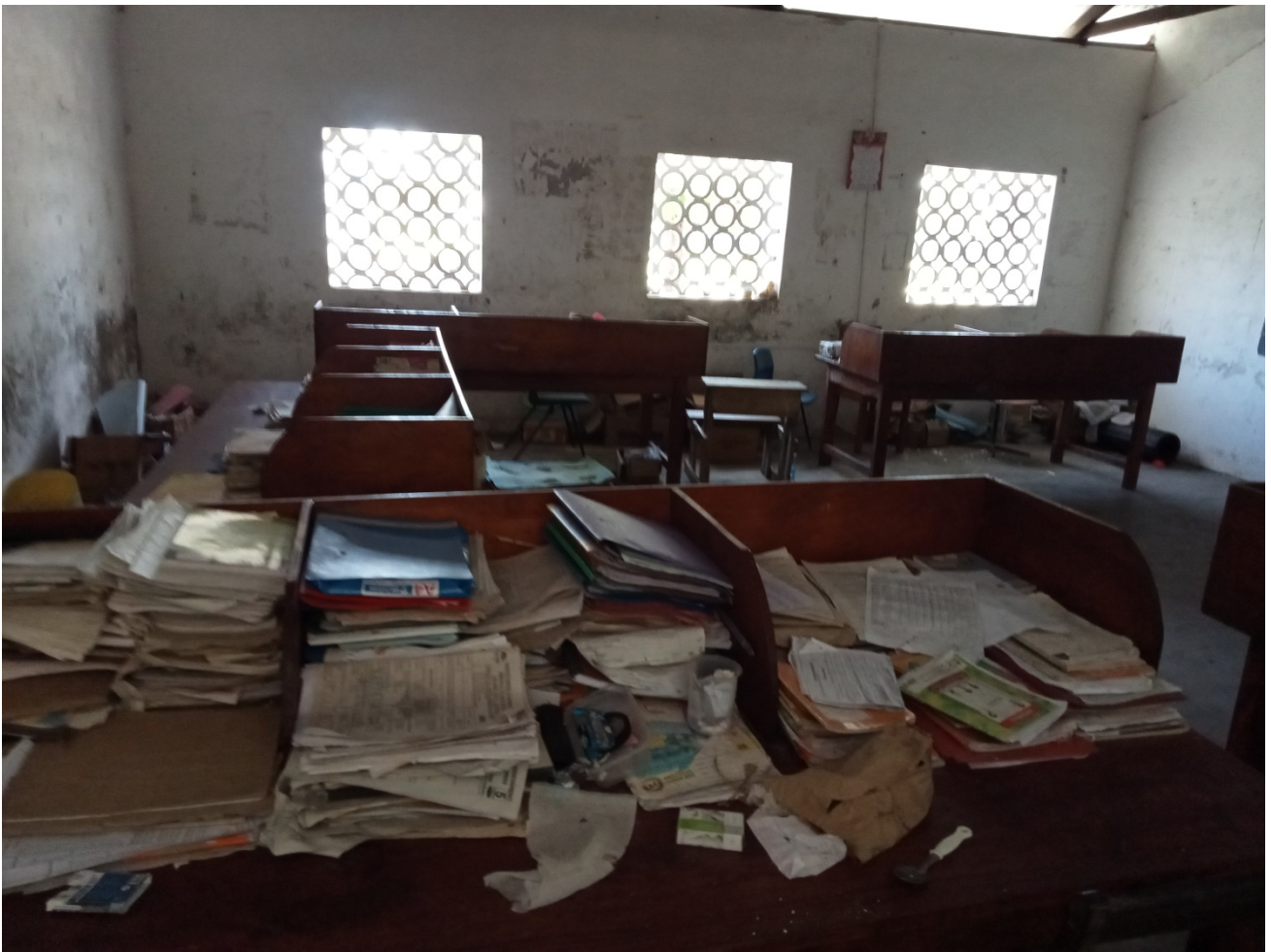
Picture ix: staffrooms are also dark even with white paint, needs 2 translucent/skylight sheet to let in natural light, the windows system do not let in enough light
